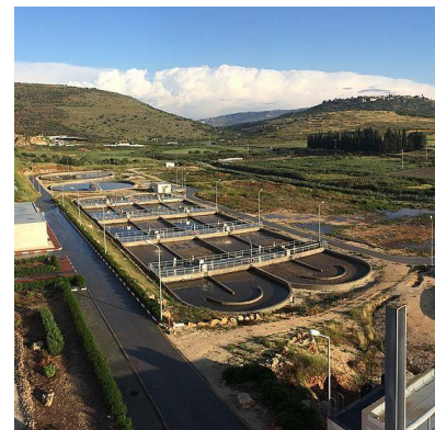
WWTP Nablus West
